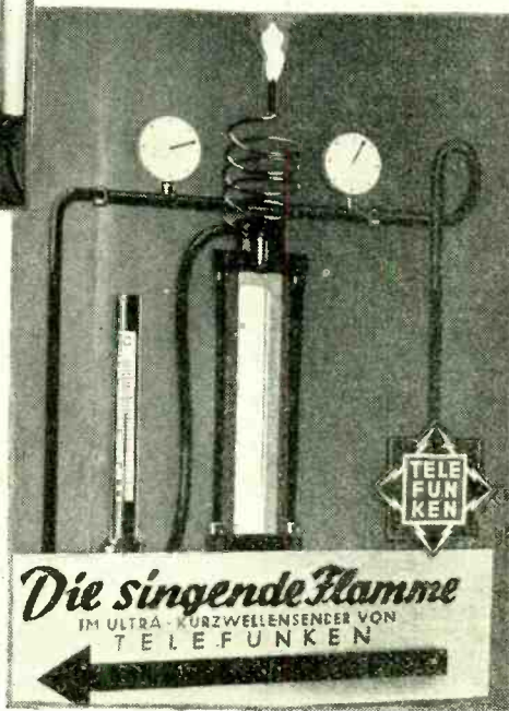
The singing flame which shows the modulation of the ultra-short-wave transmitter.
